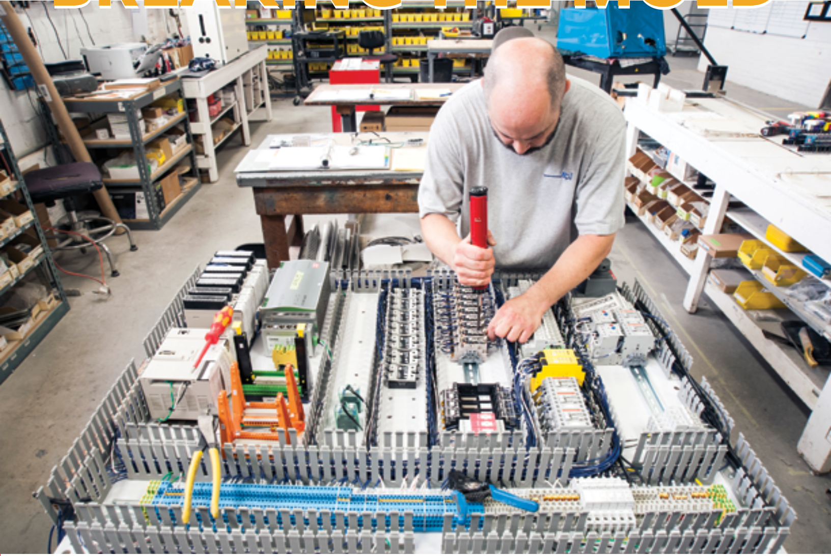
Dominic Cocco is wiring an electrical panel.
